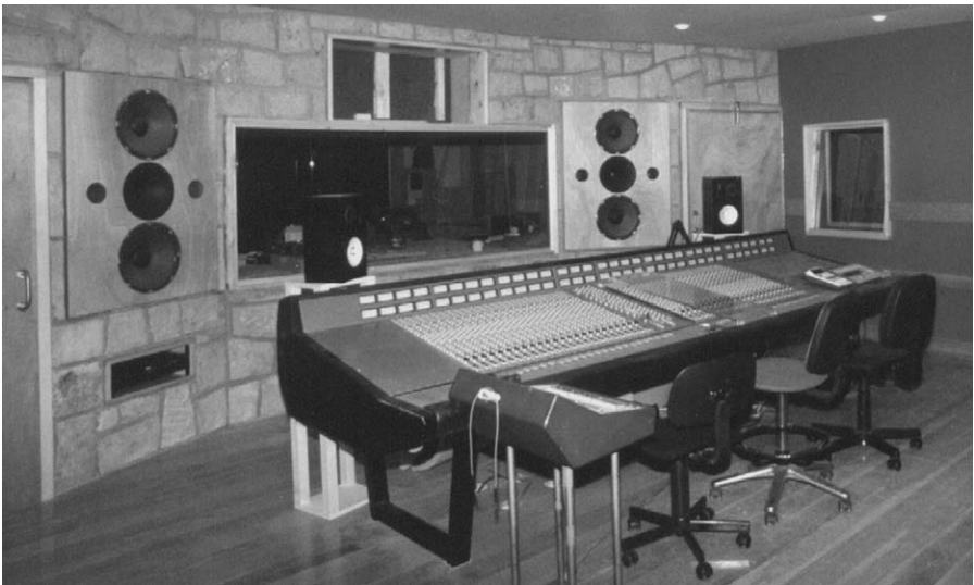
Figure 11.6. Large studio control room with main monitors utilizing round axisymmetric waveguide horn with low-frequency drivers in over/under, D'Appolito configuration. Near-field monitors are visible on stands behind console. (Courtesy Reflexion Arts.)
