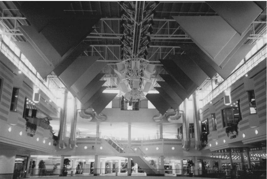
Figure 10.15. Large CD horn cluster covering indoor ice rink (Courtesy Peter Mapp Associates).
